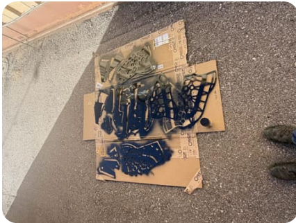
Painting CNC'd structural parts
